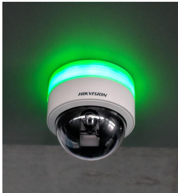
Figure 14: Jinhui OCR camera marking a vacant spot
