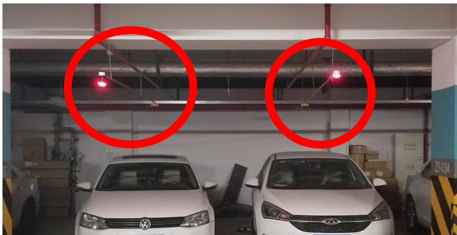
Figure 18: LED lights and ultrasonic proximity sensors observed at Huawei
