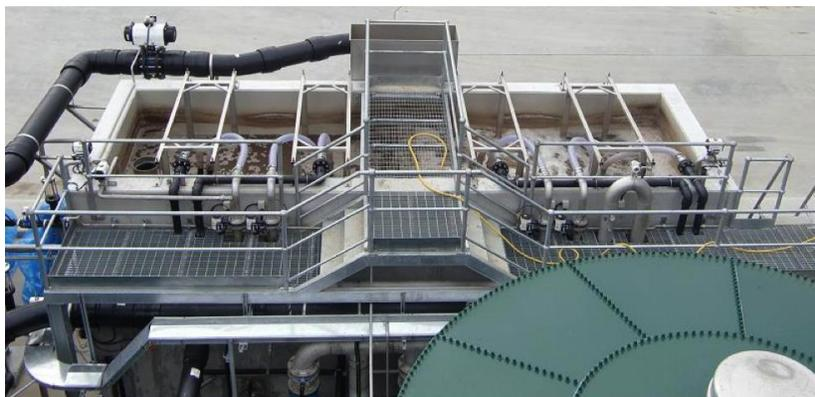
Figure 5: Bluetongue Brewery's aerobic membrane bioreactor post-treatment stage. Water in this stage is aerated in a mixing tank to supply oxygen to the microorganisms (CST Wastewater Solutions, n.d.).
