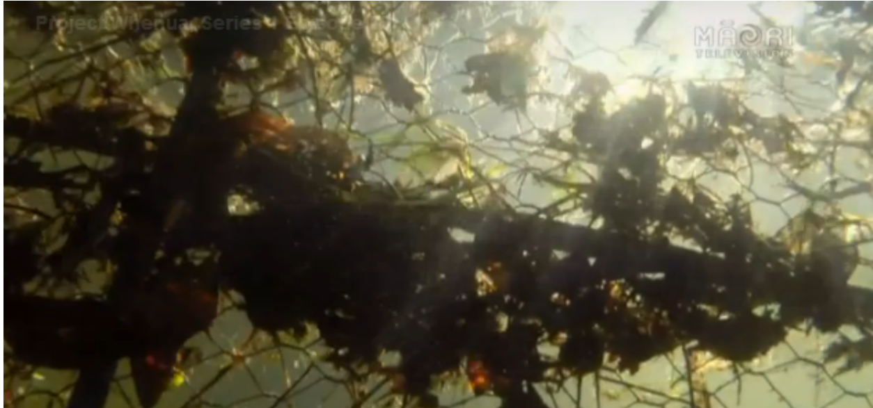
Figure 4: Underwater View of Intake Grate Congestion (Maori Television)
