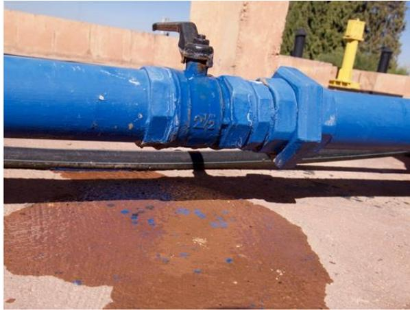
**Figure 4-18: Leaking Pipe at Water Filtration Station**
