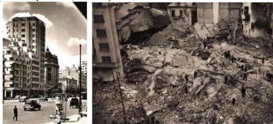
*Figure E.1: The Carlton building before and after collapse from the 1940 earthquake in Bucharest. Georgescu and Pomonis (2012).*
