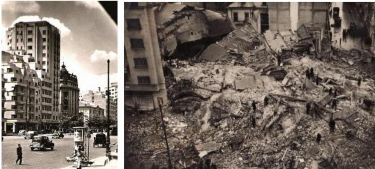
*Figure 2.9: The Carlton Block before collapse (left) and after collapse (right). Georgescu, E & Pomonis, A (2012).*
