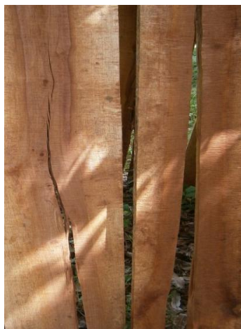
Figure 4.2- 10: Cracks in Plantation Pochote Timber
