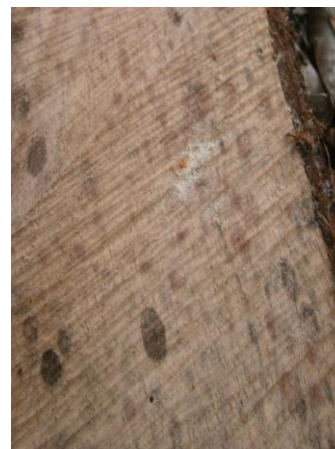
Figure 4.2- 11: Damage of Untreated Plantation Pochote Wood
