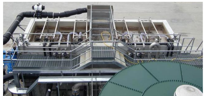
Figure 6: Bluetongue Brewery's aerobic membrane bioreactor post-treatment stage. Water in this stage aerates in a mixing tank to supply oxygen to the microorganisms (CST Wastewater Solutions, n.d.).
