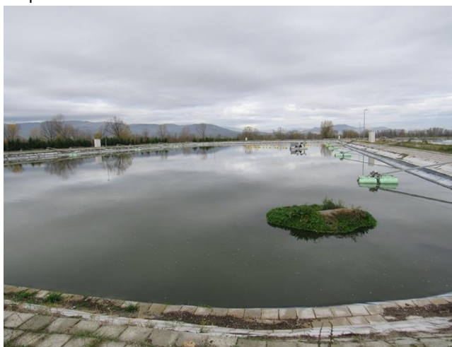
Figure 23: An aeration pond at Korçë WWTP. Taken on Nov. 15, 2019.
