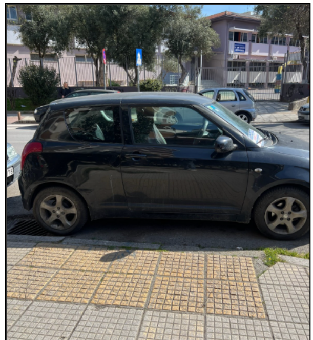
Figure 0.4: Car Blocking Curb Ramp and Tactile Slabs on the Corner of Distomou and Papafi
