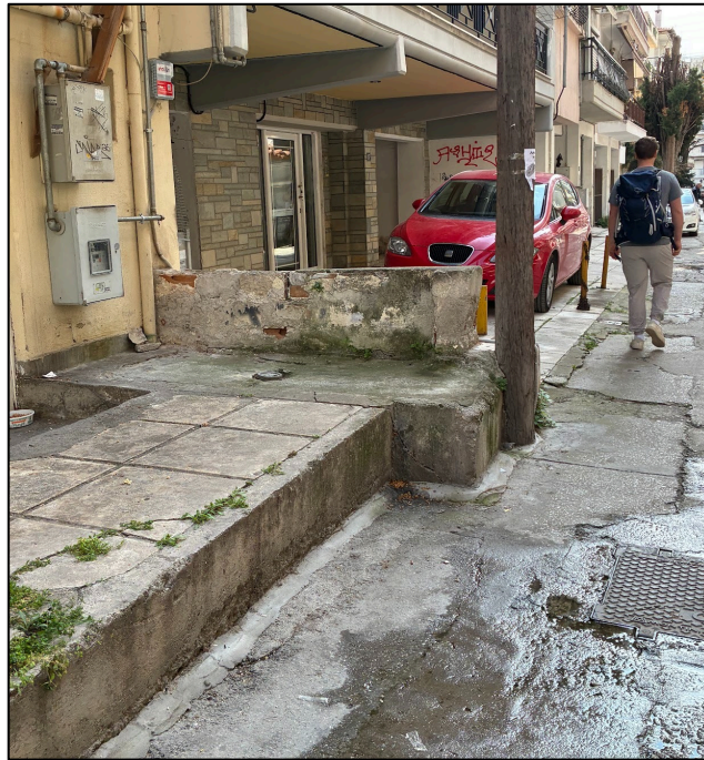
Figure 4.4: Sidewalk with Step and Blockage on Vithynias Street (near SFA center)
