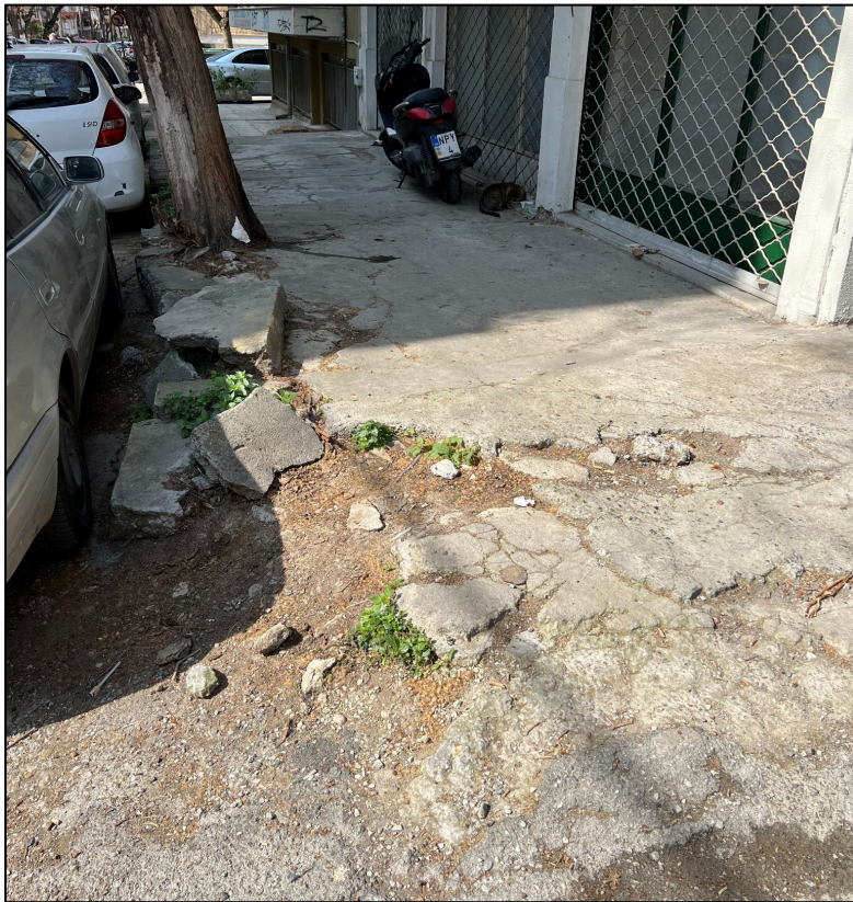
Figure 4.10: Crumbling Sidewalk and Curb on Thessaloniki – Kato Toumpa
