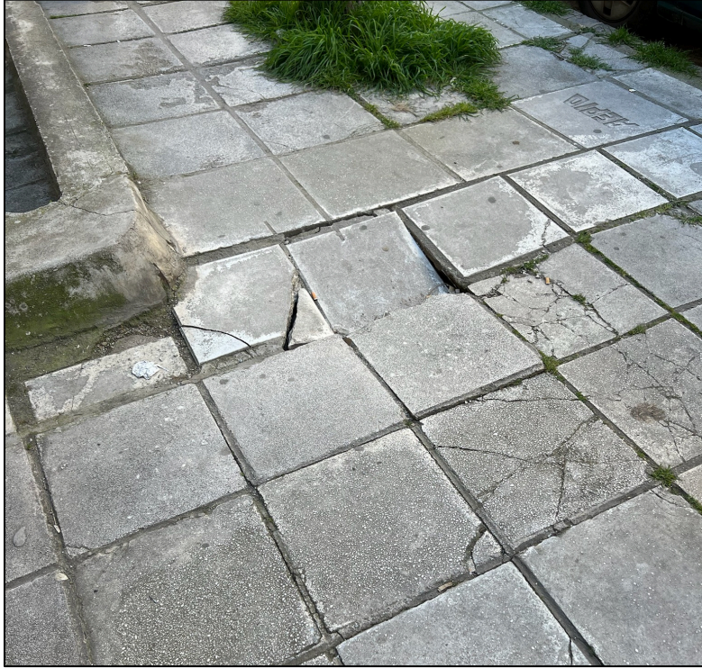
Figure 4.9: Cluster of Broken Sidewalk Tiles on Michail Chourmouzi
