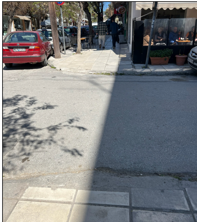
Figure 4.8: No Crosswalk and Tactile Slabs at the Intersection of Markou Botsari and Ionias
