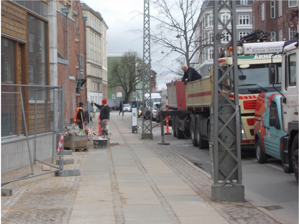
Figure 7.1.c: Large construction vehicle at Vibehus Skole.
