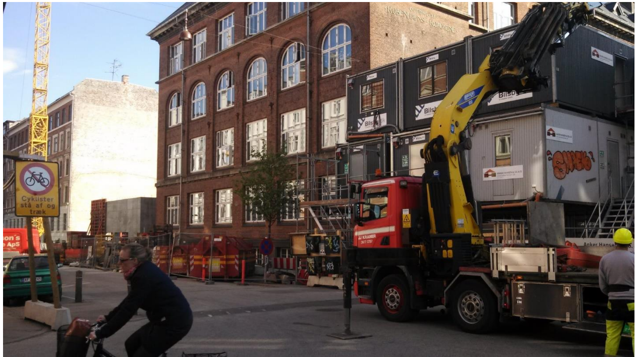
Figure 6.1.c: Langelinieskolen with visible, active construction next to school
