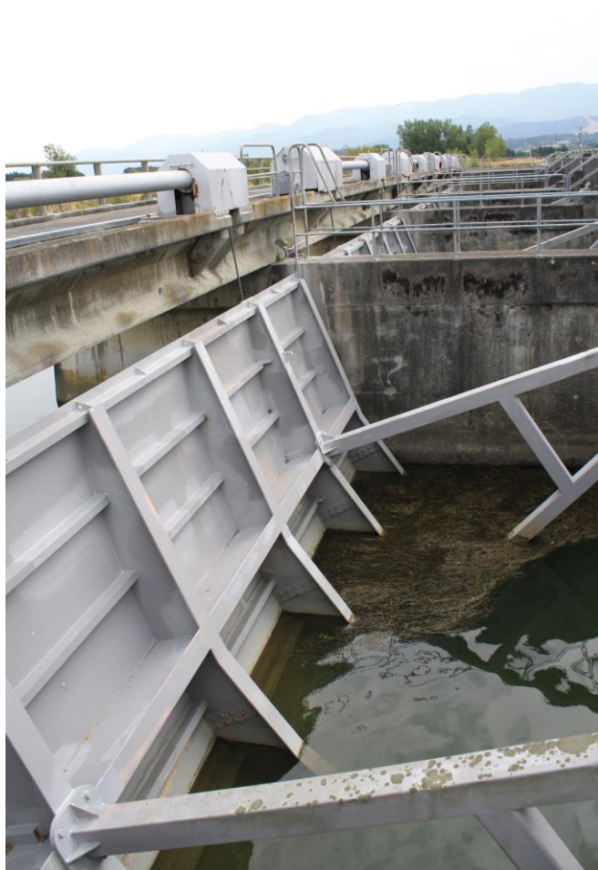
Figure 15 - The Blundell Barrage Gates: top view
