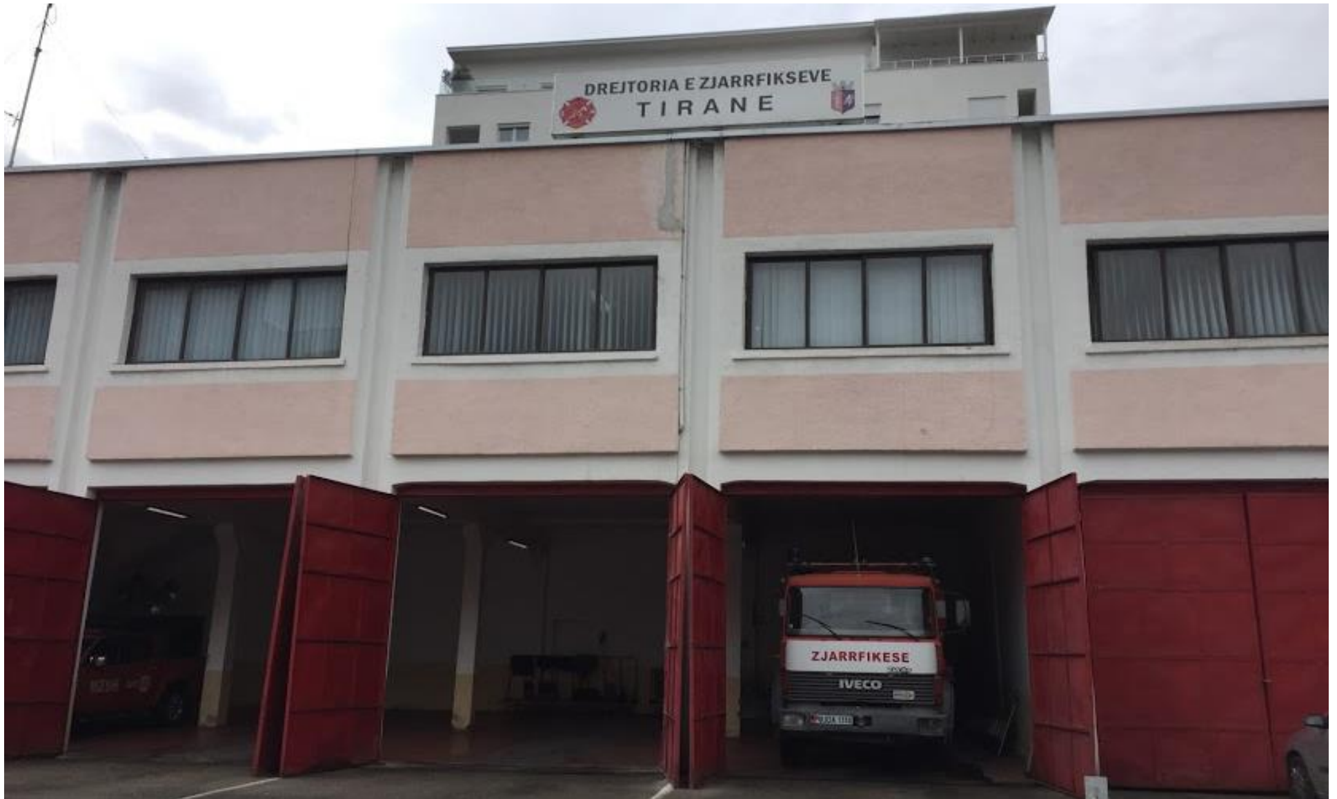
Figure 27: Main Fire station in Tirana
