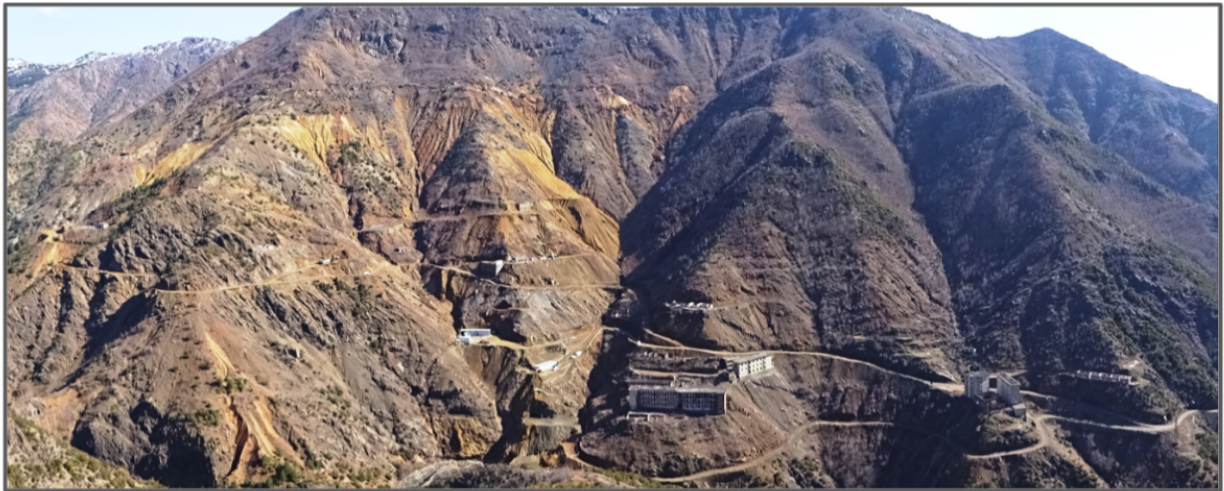
Fig 1.1 Full Site View of Spaç in 2017 (Courtesy of CHwB)
