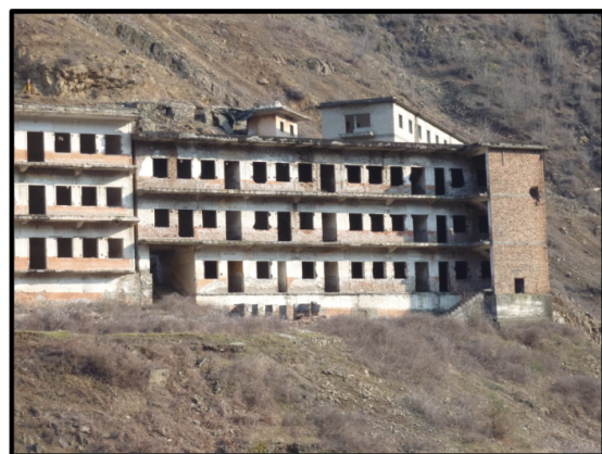
Fig 1.2 NW Facade (Courtesy of CHwB)
